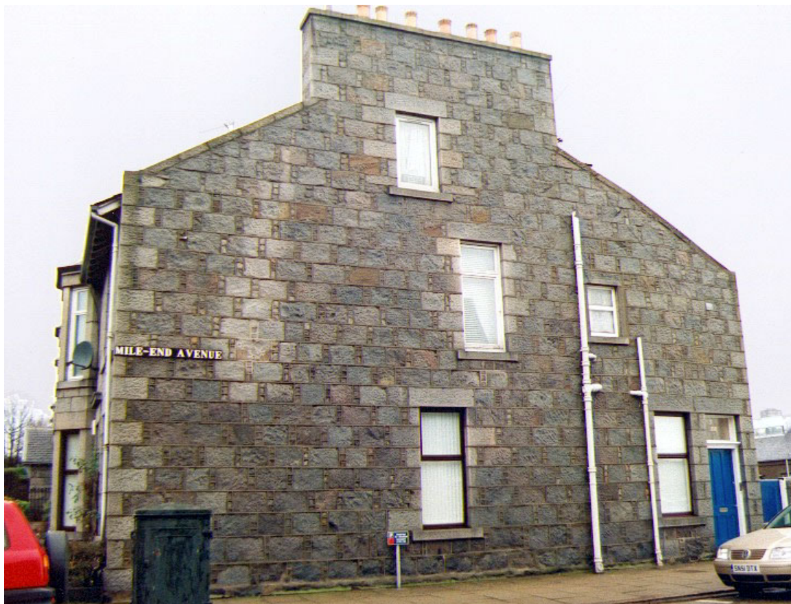
Plate 2.4 The irregularly distributed windows on this gable have projecting cills. Downpipes also project from the surface. The dry patch towards the left side is likely to indicate the presence of a working fireplace.
