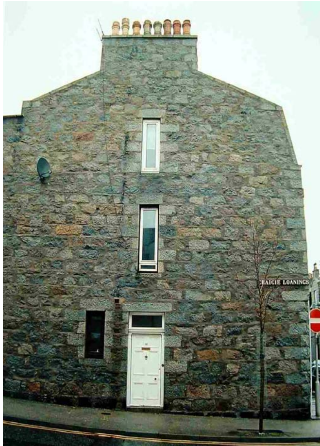
Plate 2.4 The irregularly distributed windows on this gable have projecting cills. Downpipes also project from the surface. The dry patch towards the left side is likely to indicate the presence of a working fireplace.
