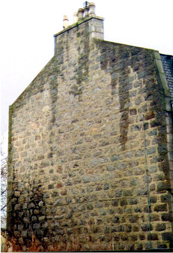
Plate 2.1 Typical, simple granite gable. Three storeys in height with no detailing except a slightly projecting coping at the top of the chimney. This gable shows a typical wetting pattern from moderate rainfall with wetting of chimney, wall tops and corners. Run-off from these areas gradually extends down the gable.
