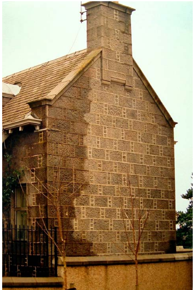
Plate 2.6 The projecting chimneys on this façade (which in this instance were directly facing the wind driven rain (2 knots)) have clearly influenced the impact of rain on the façade. Wind flow has been slowed by the projecting features.
