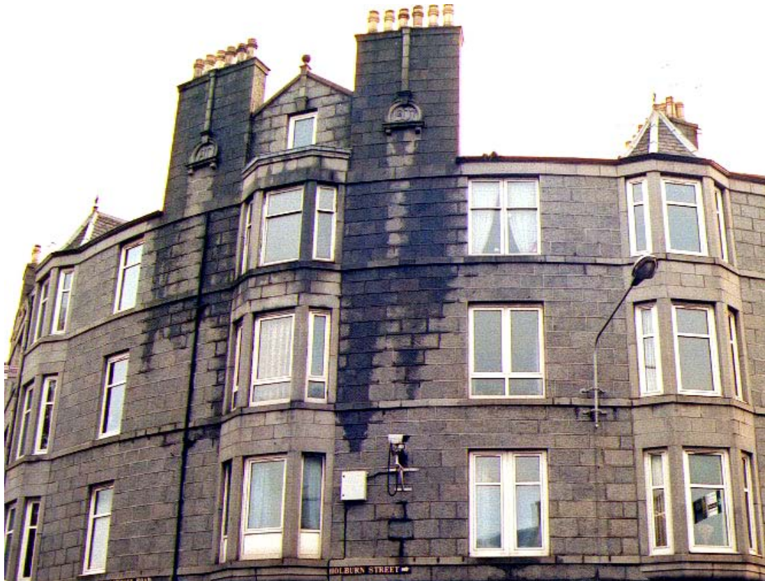
Plate 2.6 The projecting chimneys on this façade (which in this instance were directly facing the wind driven rain (2 knots)) have clearly influenced the impact of rain on the façade. Wind flow has been slowed by the projecting features.
