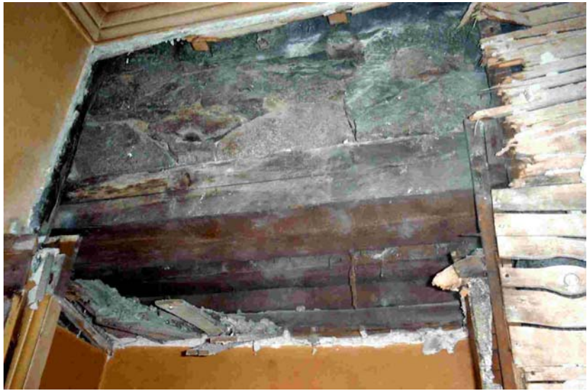
Plate 4.6 Stripping internal wall. Wall and timber safe lintel above alcove.
