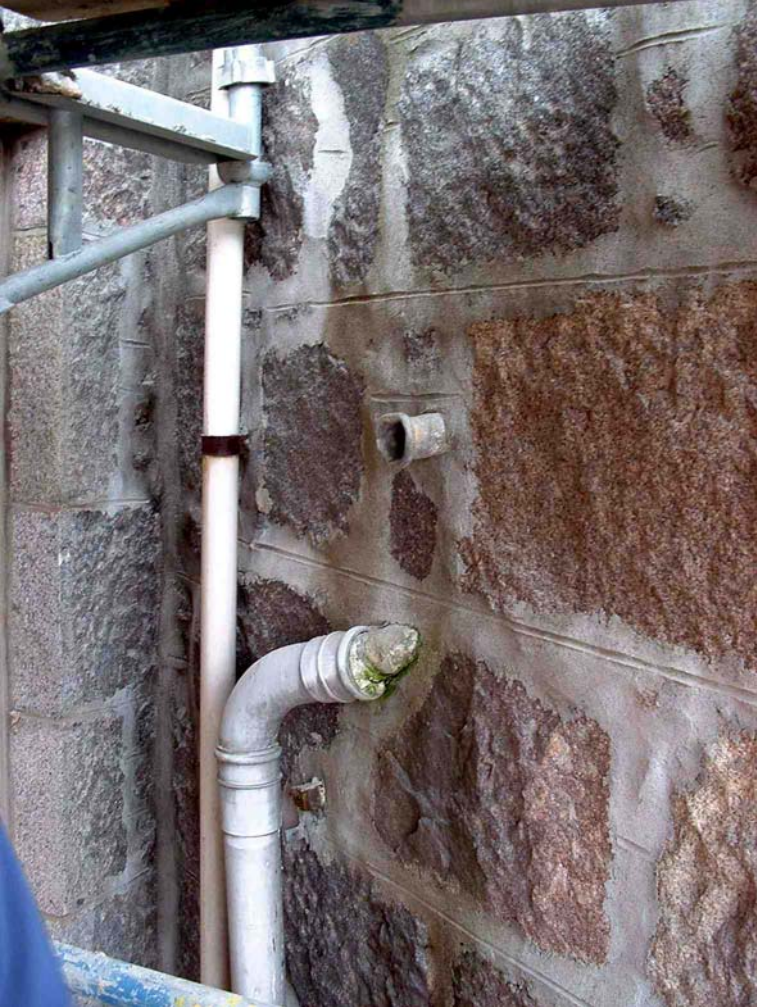
Plate 4.14 Parapet gutter and overflow after unblocking (Feb 2003).
