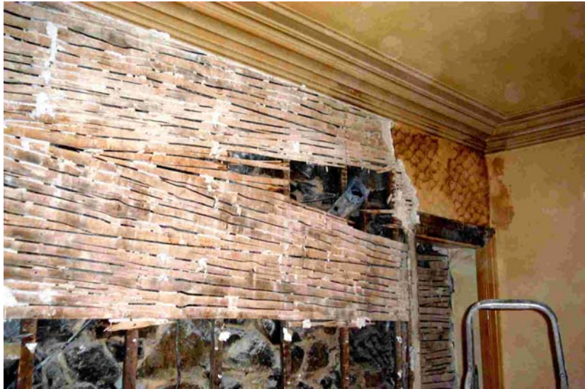
Plate 4.6 Stripping internal wall. Wall and timber safe lintel above alcove.
