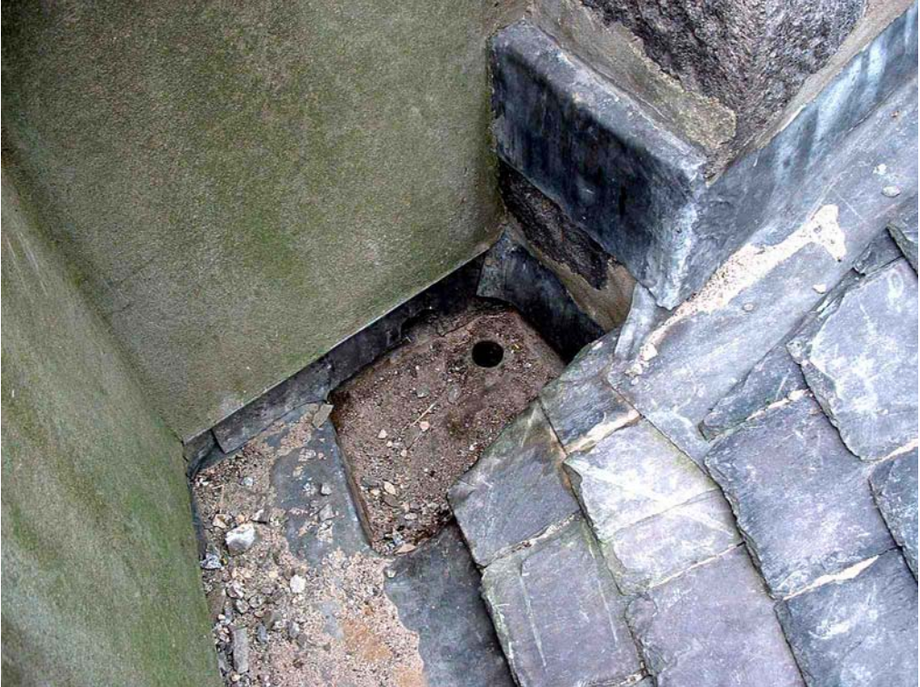
Plate 4.14 Parapet gutter and overflow after unblocking (Feb 2003).
