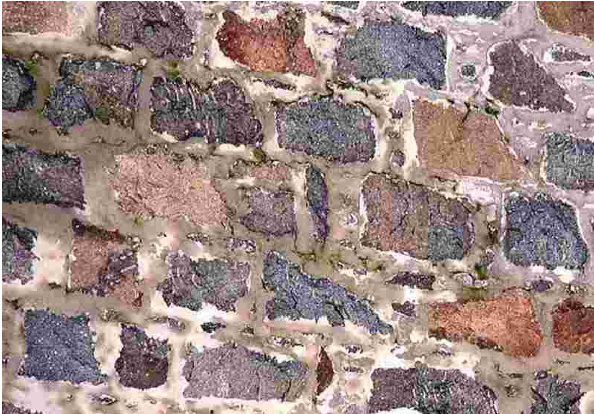
Plate 4.31 Damp pointing (darker area) on the front façade with green algal growth (photographed in March 2003).
