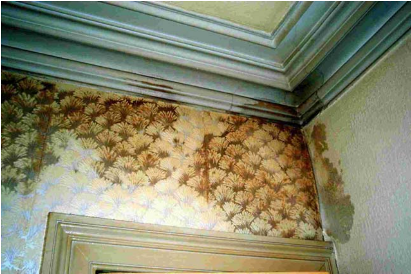
Plate 4.5 Stripping internal wall.
