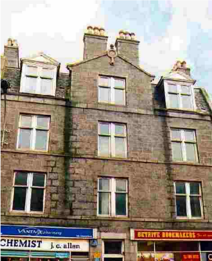
Plate 4.7 Front facade of case study two showing green algal growth on area affected by rainwater run-off.
