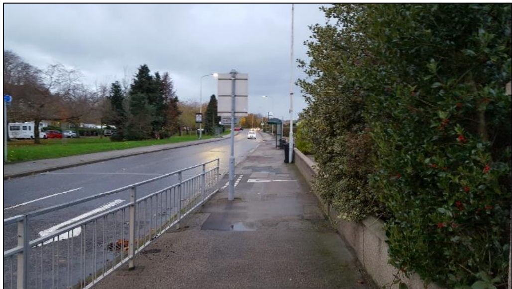
Footway on Inverurie Road
