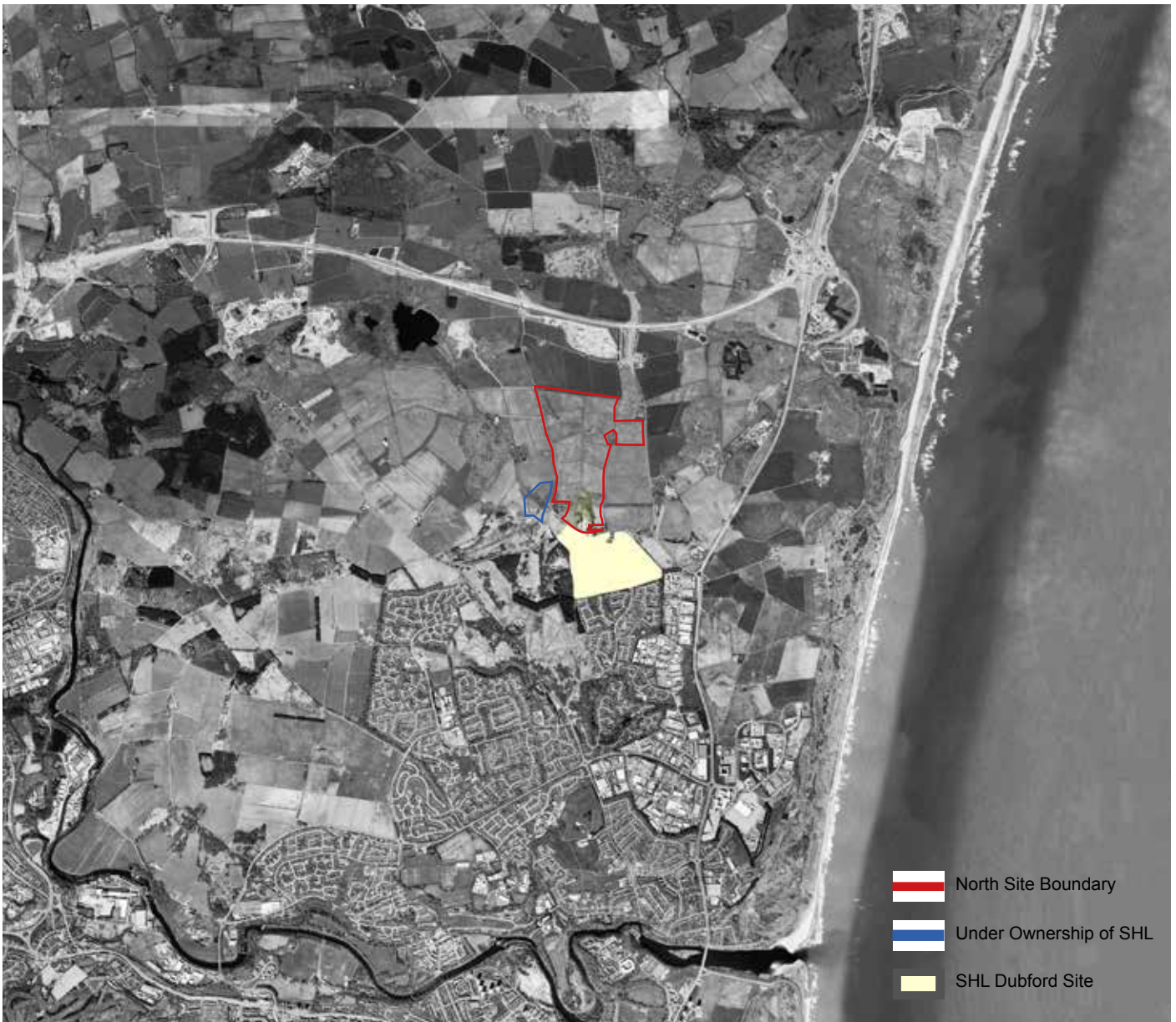
Aerial Photograph showing Site Context & Completed Dubford Development to the South
