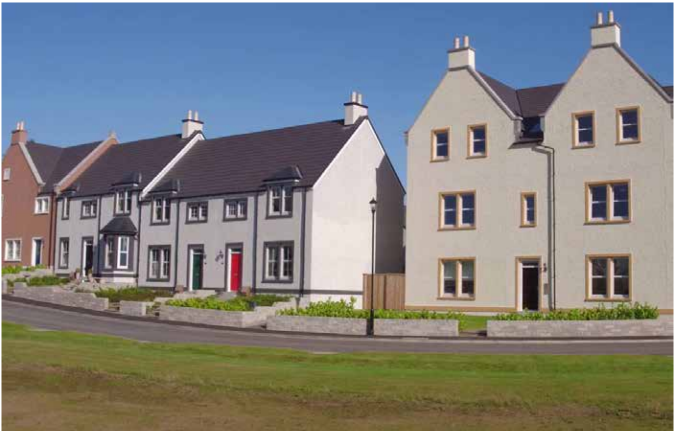
Scotia Homes existing development
