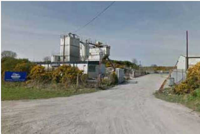
Existing Concrete Plant / Quarry Entrance
