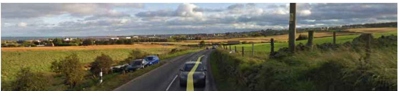
View of B999 looking south
