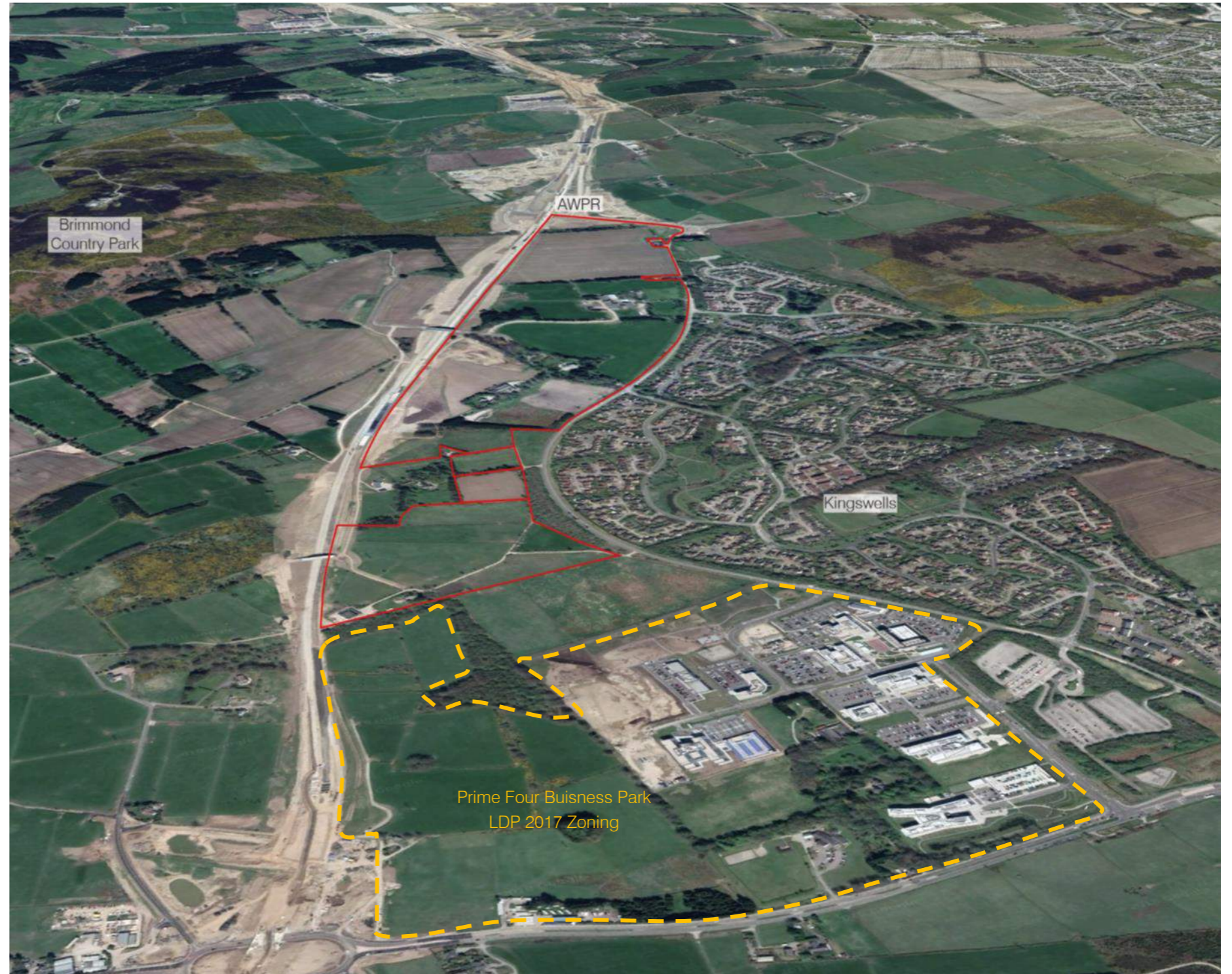
Aerial View of AWPR Works
