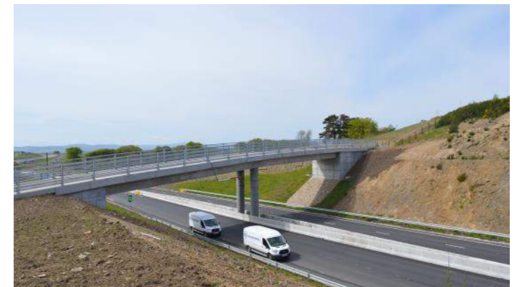
Photograph of the footbridge over the AWPR (south west corner of site)
