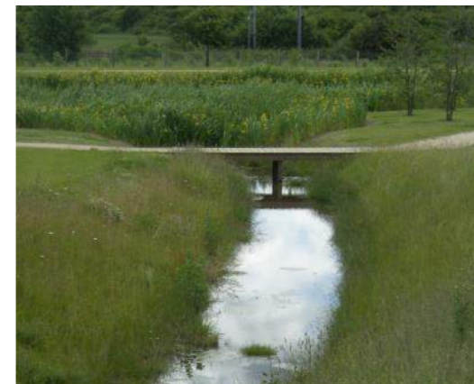
Swale pond surrounded in soft wetland vegetation as proposed for integrated SUDS ponds.
