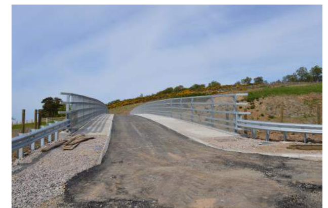
Footpath connections lead to pedestrian bridge over AWPR
