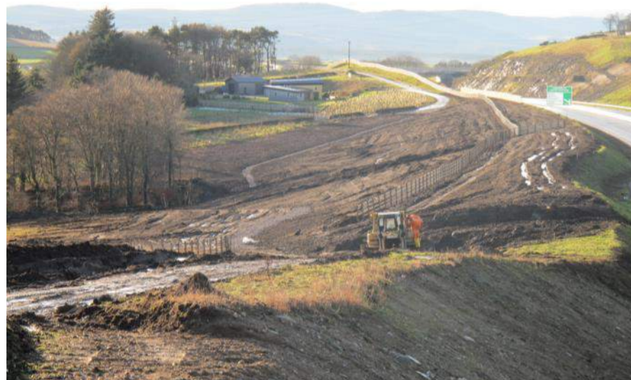
Photography of AWPR Works at Site Boundary
