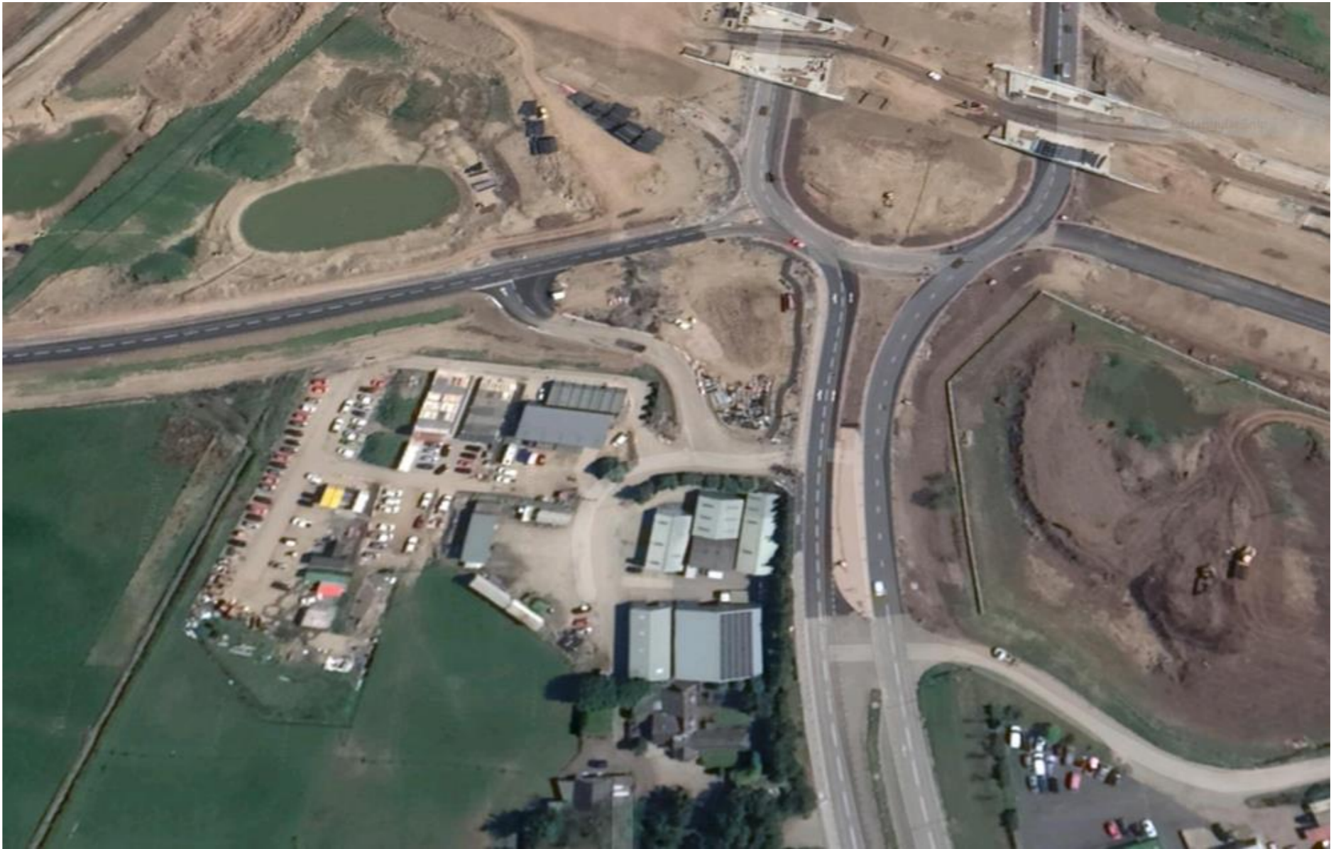
The site from the west (Google Maps)
