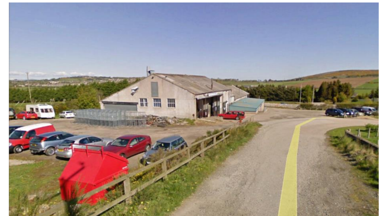
Southern elevation of the existing commercial unit
