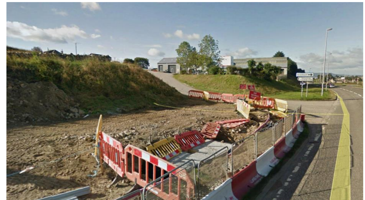
View to the site from A944—note existing access
