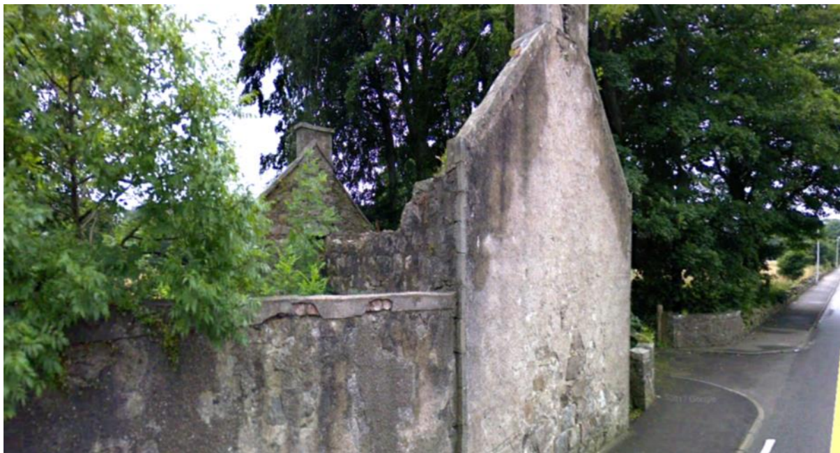
The redundant steading building to the North of the site - (Source: Google Maps)
