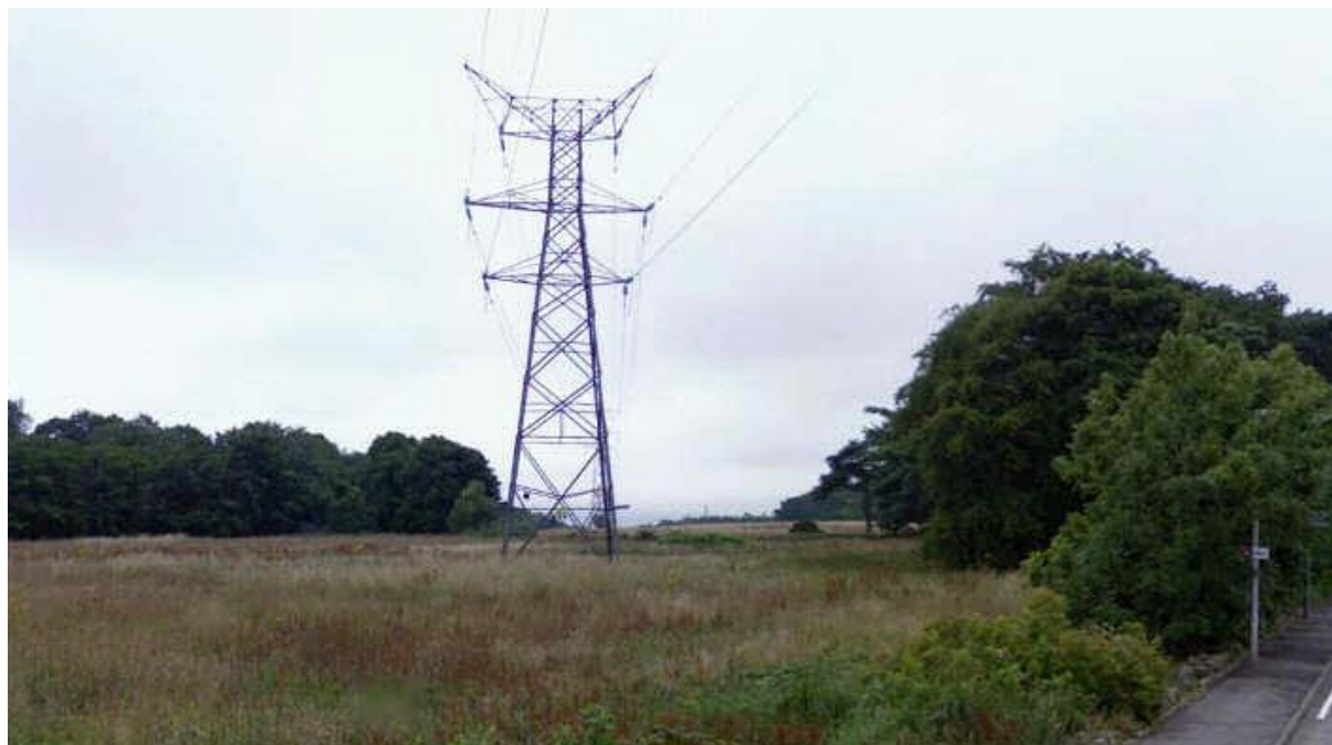
Pylons to the north of the site- (Source: Google Maps)
