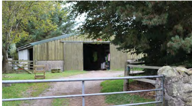
Stable buildings within the site area.
