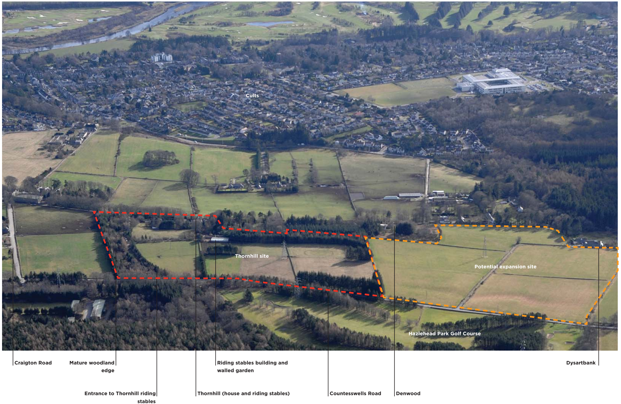
Fig. 02: Aerial view of site from north.
