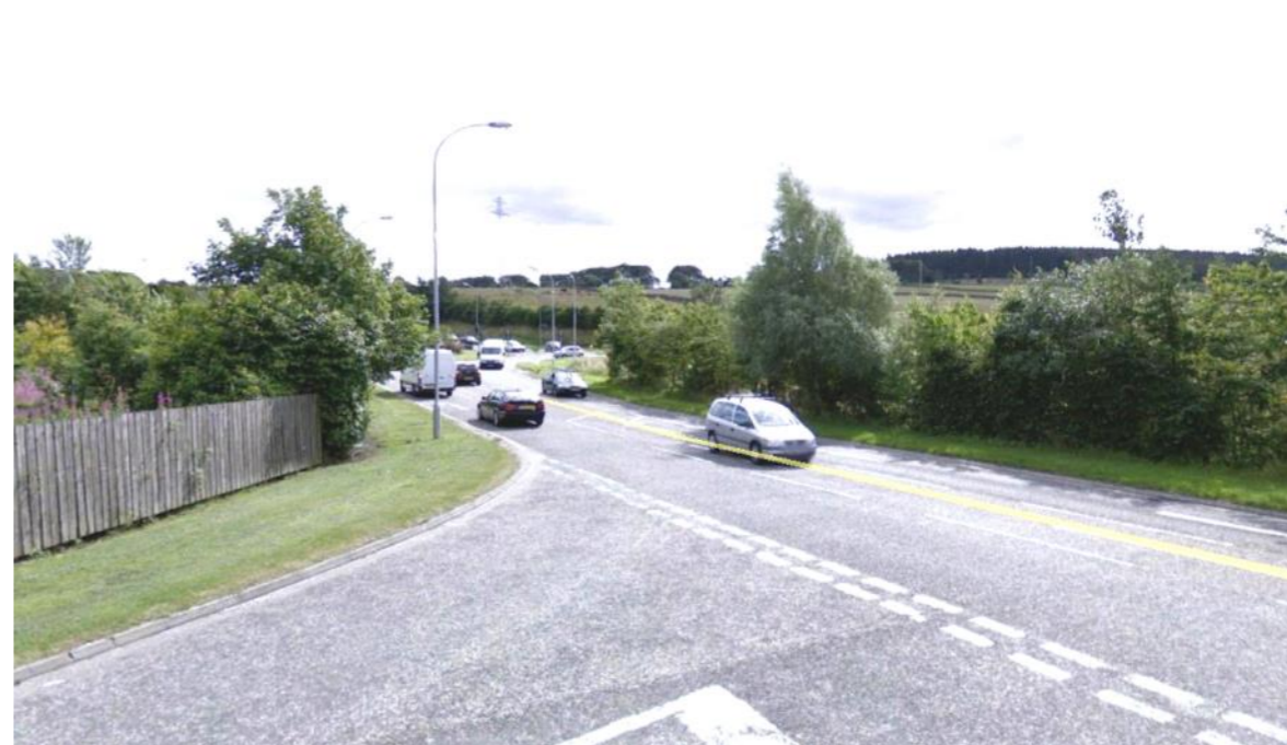
Site viewed from north— note woodland backdrop to south
