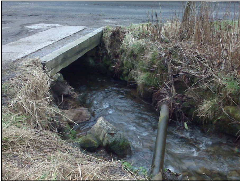
Photo1: View of the Sunnyside culvert inlet from within the site
