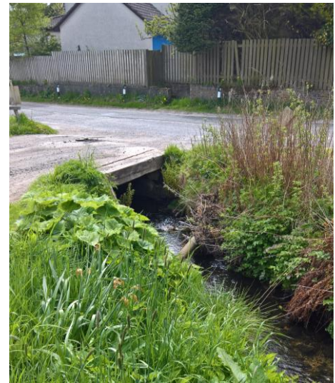
Figure 9: Existing Crossing at Sunnyside
