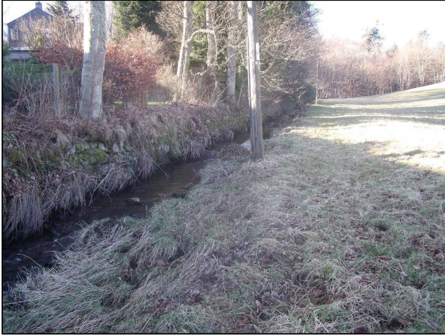
Photo 3: View looking west, upstream, along the southern site boundary from the Sunnyside culvert
