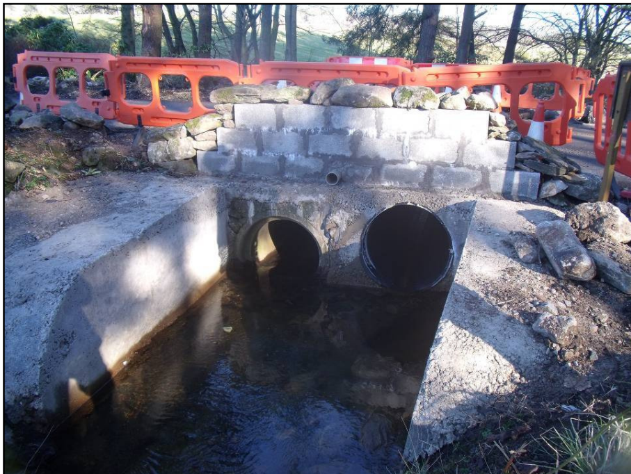
Photo 2: View of the upstream face of the Craigbank culverts
