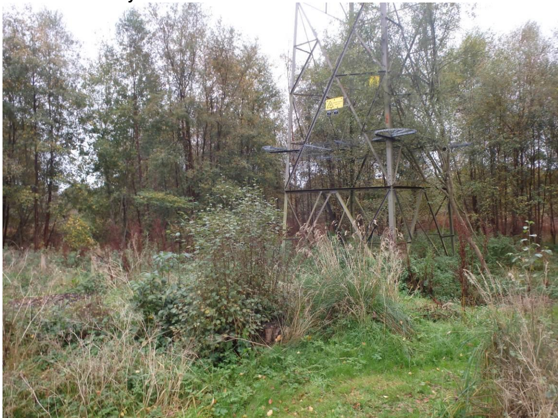
Photo 8: Electricity Pylon within central field
