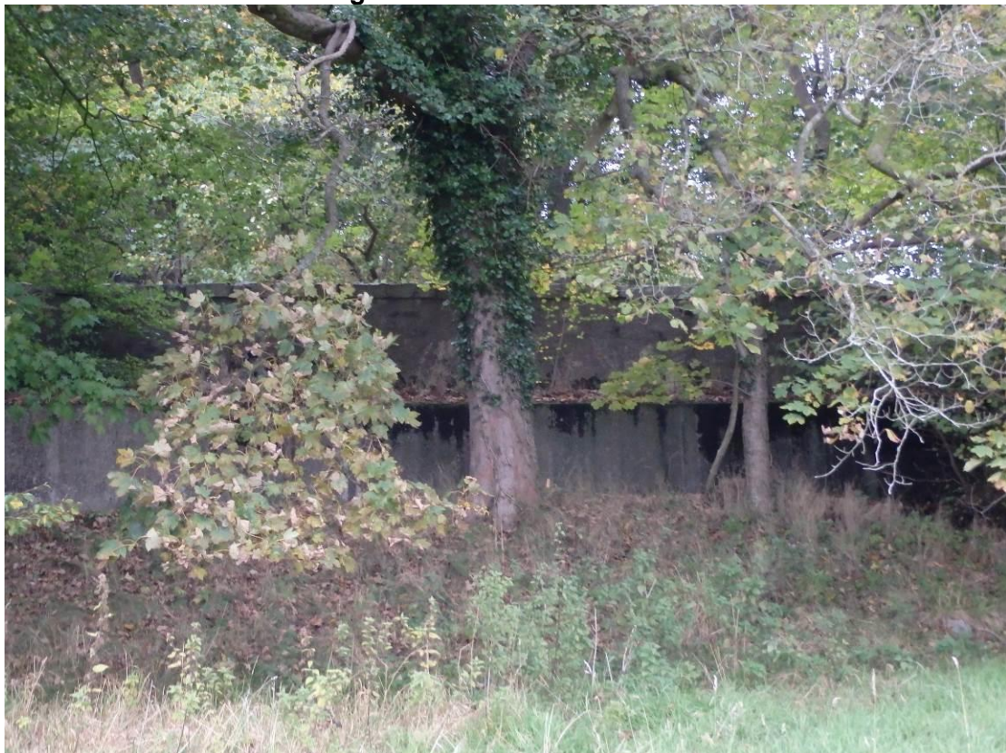
Photo 12: Potential retaining wall in north west of northern field
