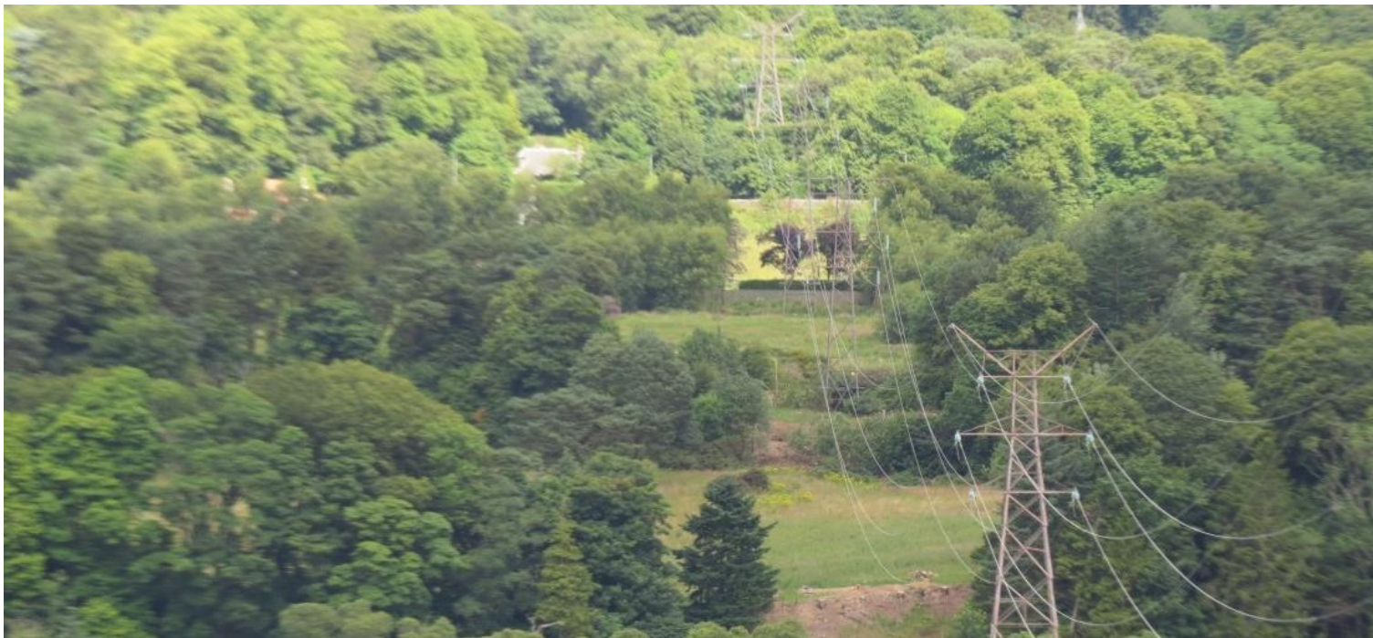
Photo 19a: Close up of photo 10. View of application site. The only views are along the pylon wayleave. The views of the site are mainly prevented by the mature trees in the ancient woodland along Inchgarth Road. From these areas of Deeside, the application site is distant with many areas with limited views to the application site. The open areas of the site seen in this photograph are retained as open areas with new tree planting forming wildlife corridors.
