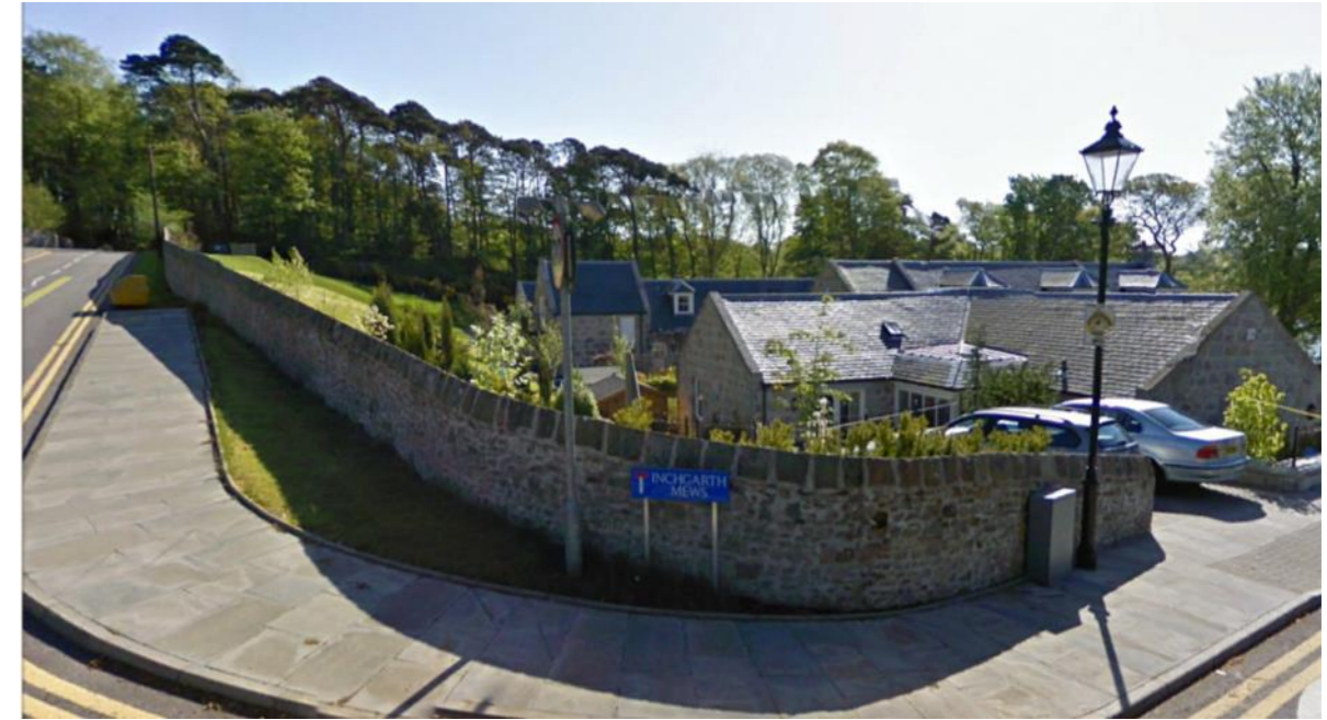
The existing residential development to the west- (Source:Google Map)
