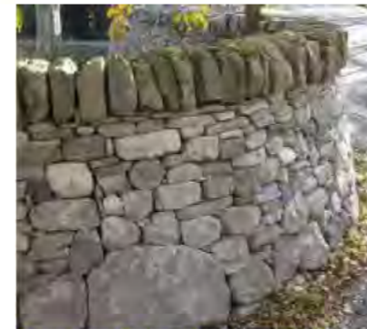
Drystone Dyke / Feature Walls
