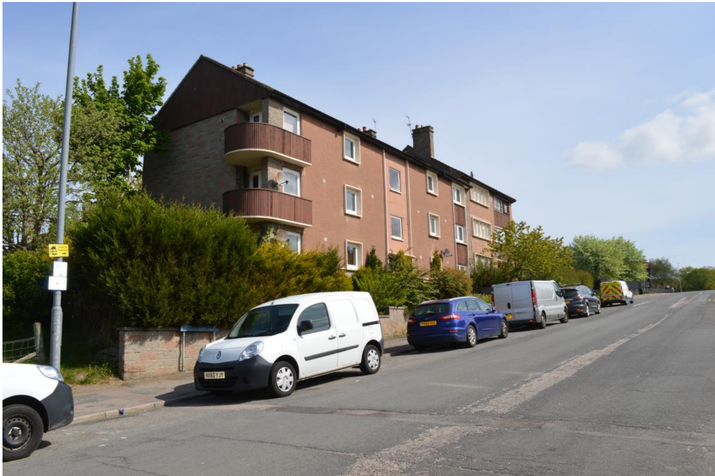
Adjacent flats on Auchinyell Road
