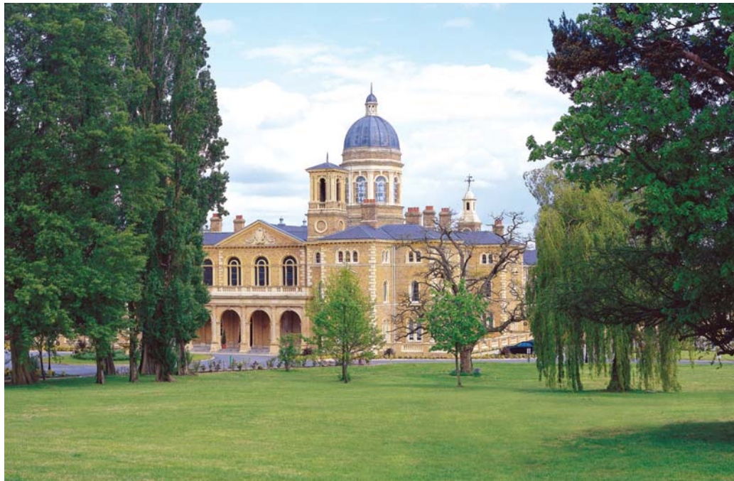
Princess Park Manor, Friern Barnet, North London Residential Masterplan of Listed Estate Project Stage: Complete
