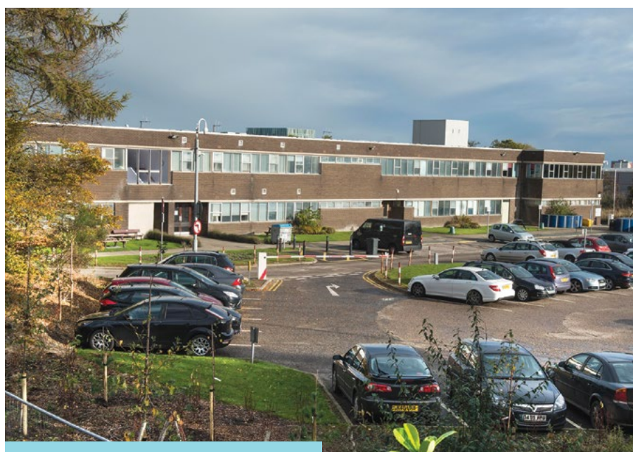
Views of Building Services at Kittybrewster
